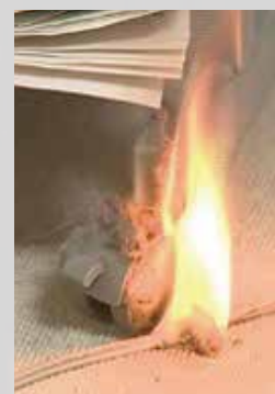
Fire from a partly broken wire
