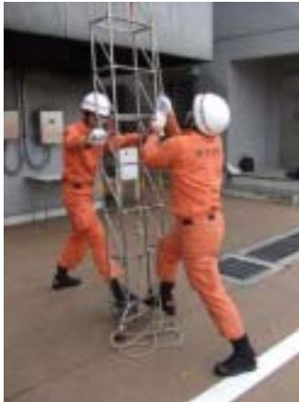
Photo 5: Handling of 3-Extension Ladders
